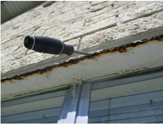
25 Right Side of Building Lintel Sag w/ Severe Corrosion
