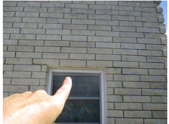
12 Front Right Lintel Sag w/ Severe Corrosion
