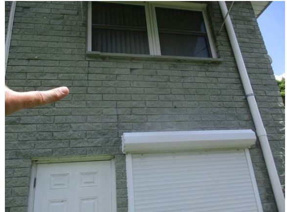
44 Rear of Building Fluted Block Cracked Between 1st & 2nd Floors
