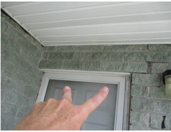
9 Unit #12 Lintel Sag w/ Fluted Block Cracking
