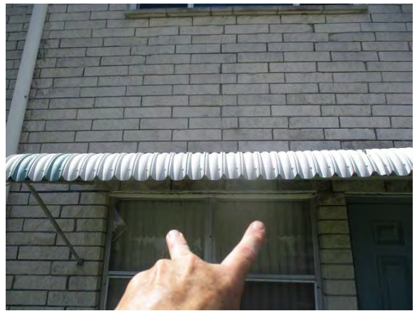
38 Rear of Building Lintel Sag w/ Severe Corrosion
