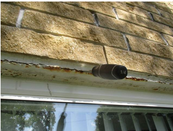
23 Right Side 1st Floor Lintel Severe Corrosion
