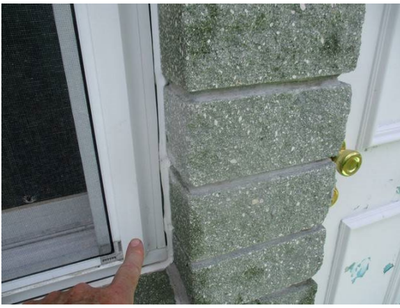
33 Window Caulking Deteriorated/Missing Throughout
