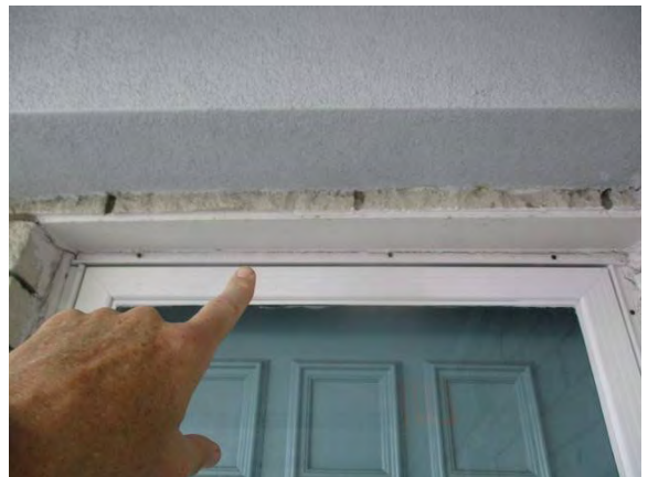
8 2nd Floor Walkway Lintels Minor Corrosion
