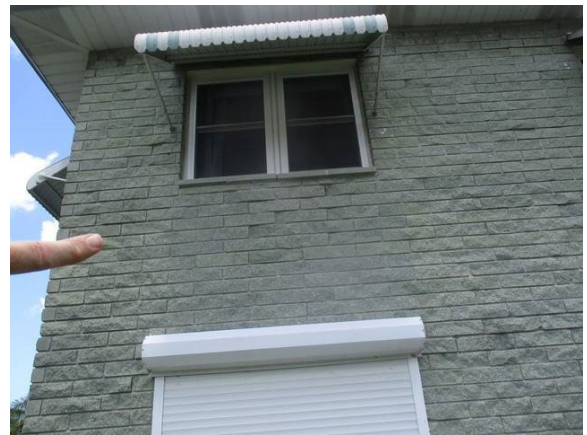
46 Left Side of Building Fluted Block Cracked Between 1st & 2nd Floors
