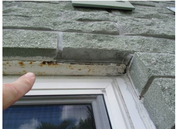
12 Front Right Lintel Sag w/ Severe Corrosion
