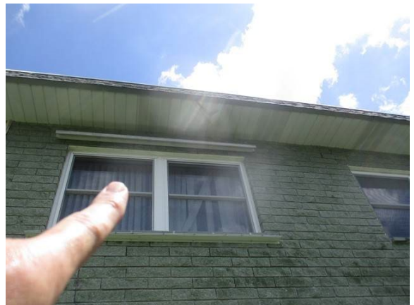
32 2nd Floor Lintels Minor Corrosion
