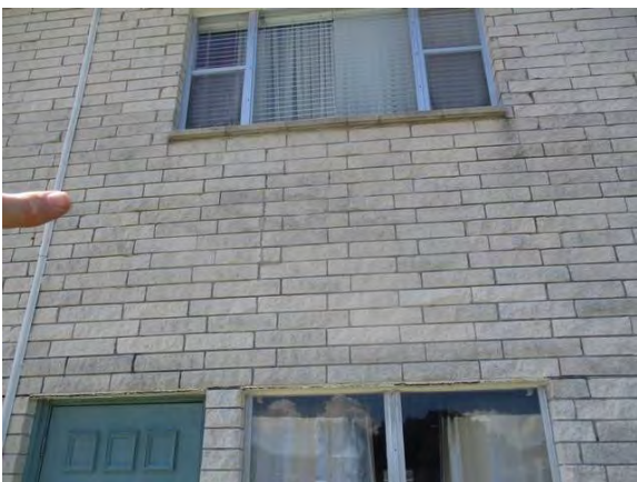
47 Rear of Building Fluted Block Cracked Between 1st & 2nd Floor
