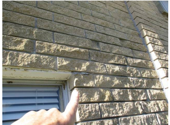
36 Rear of Building Lintel Sag/Severe Corrosion & Block Cracked
