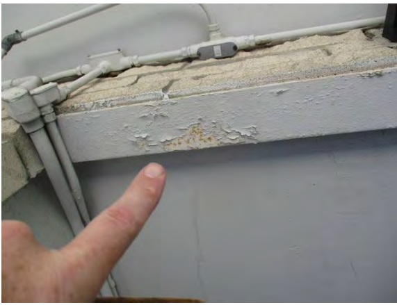
17 Hallway Lintel Minor Corrosion/Peeling Paint
