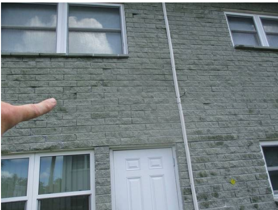
23 Rear of Building Fluted Block Cracked Between 1st & 2nd Floors
