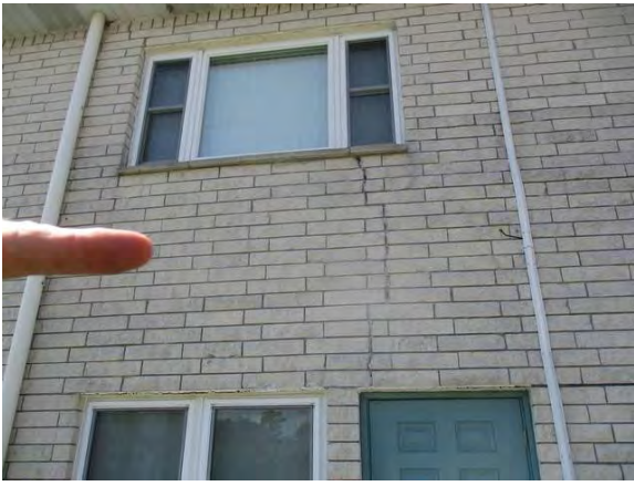
33 Rear of Building Fluted Block Cracked Between 1st & 2nd Floor
