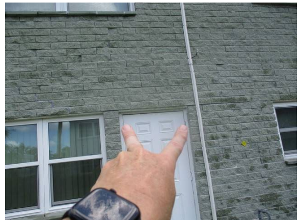
22 Rear of Building Lintel Sag w/ Severe Corrosion
