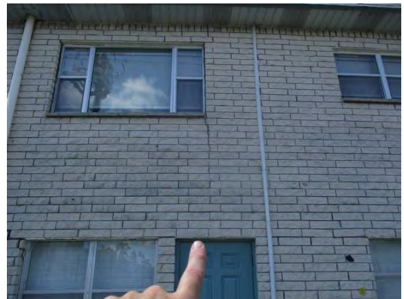
30 Rear of Building Fluted Block Cracked Between 1st & 2nd Floor
