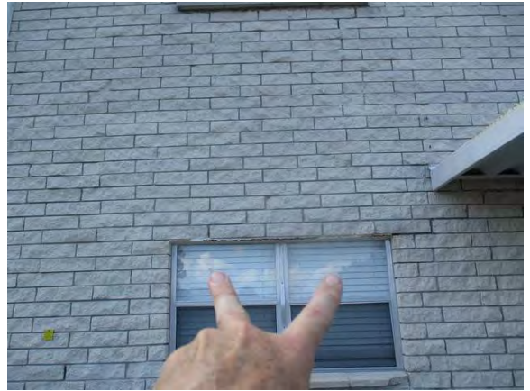
44 Rear of Building Lintel Sag w/ Severe Corrosion
