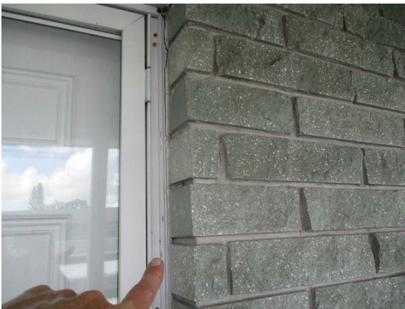
7 Door Caulking Deteriorated/Missing Throughout
