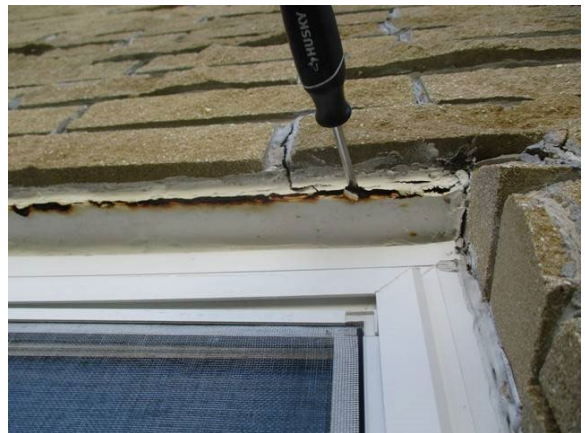
54 Left Side of Building Lintel Sag w/ Severe Corrosion
