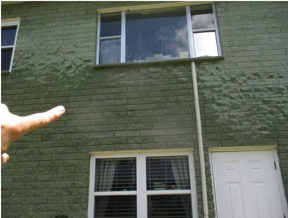
43 Rear of Building Fluted Block Cracked Between 1st & 2nd Floors
