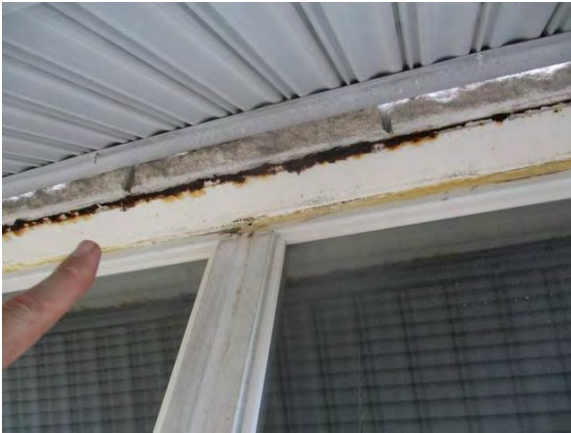
51 Left Side of Building Lintel Severe Corrosion
