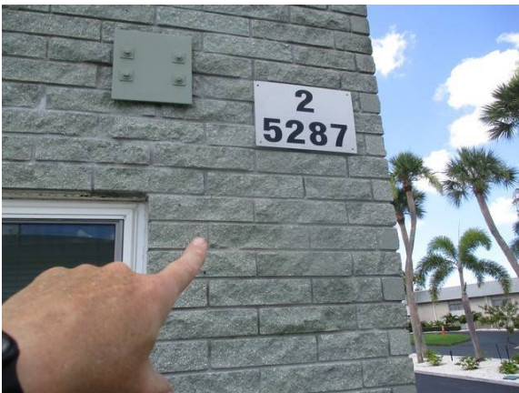
13 Front Right Fluted Block Cracked
