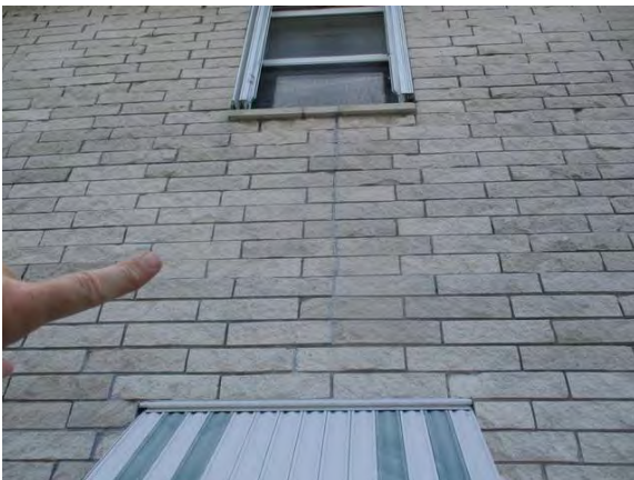
55 Left Side of Building Fluted Block Cracked Between 1st & 2nd Floor
