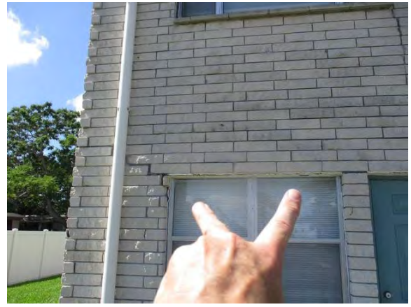
26 Rear of Building Lintel Sag w/ Fluted Block Cracking
