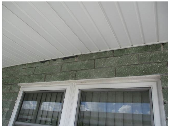
8 Walkway Lintels Minor Corrosion
