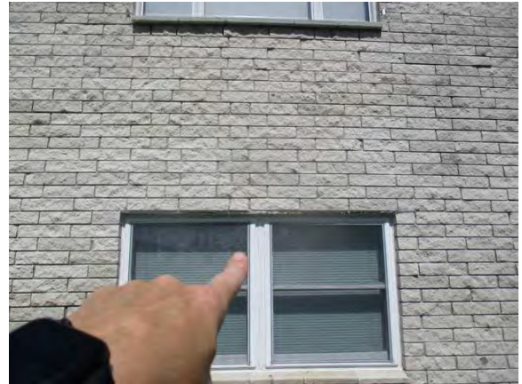
20 Right Side of Building Lintel Sag w/ Severe Corrosion
