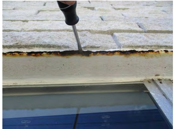
46 Rear of Building Lintel Sag w/ Severe Corrosion
