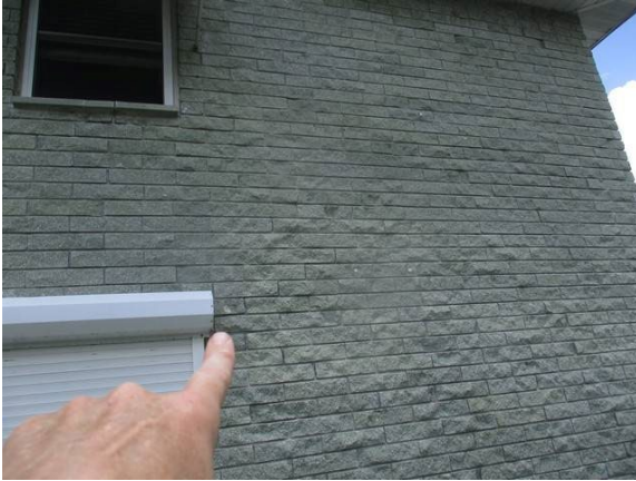
51 Left Side of Building Fluted Block Cracked Between 1st & 2nd Floors
