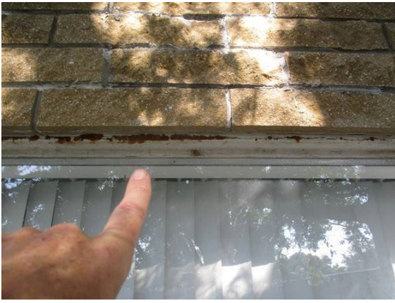
17 Right Side 1st Floor Lintel Severe Corrosion
