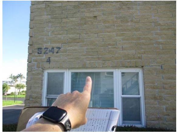
12 Front Left Lintel Sag w/ Excessive Corrosion
