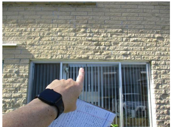
24 Rear of Building Lintel Severe Corrosion w/ Sag
