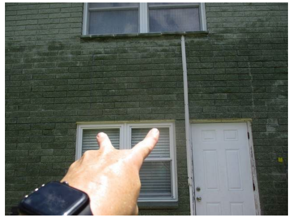
42 Rear of Building Lintel Sag w/ Severe Corrosion
