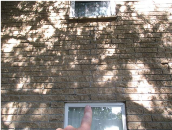
21 Right Side 1st Floor Lintel Severe Corrosion w/ Sag
