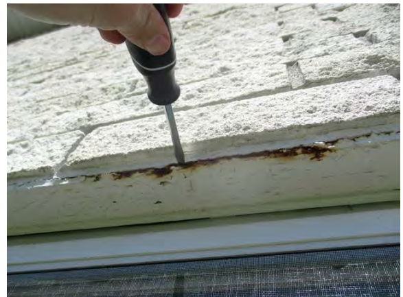
22 Right Side of Building Lintel Sag w/ Severe Corrosion
