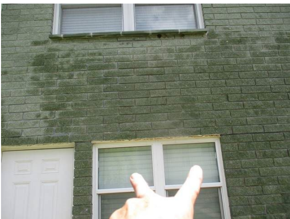
39 Rear of Building Lintel Sag w/ Severe Corrosion
