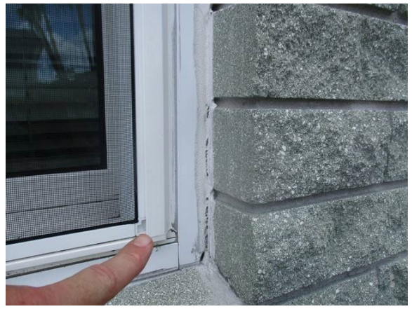
10 Window Caulking Deteriorated/Missing Throughout
