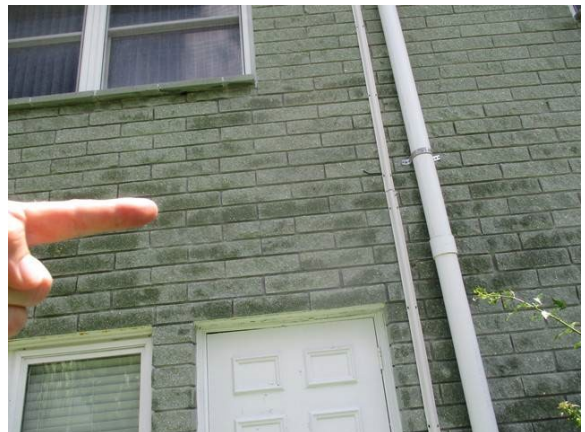
38 Rear of Building Fluted Block Cracked Between 1st & 2nd Floors
