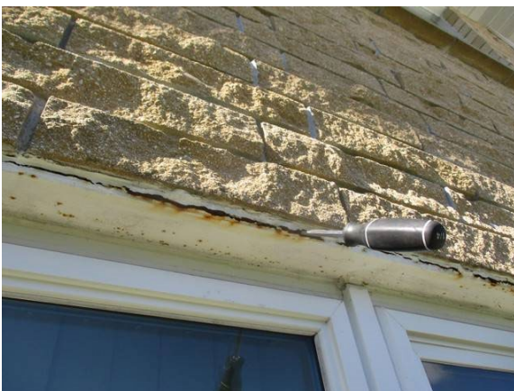
31 Rear of Building Lintel Severe Corrosion w/ Sag
