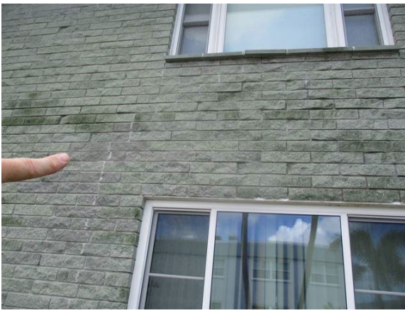
17 Right Side of Building Fluted Block Cracked Between 1st & 2nd Floors
