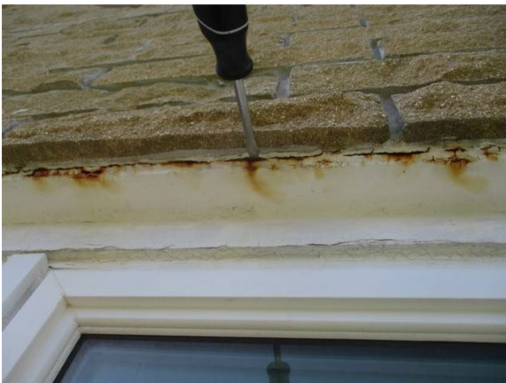
45 Rear of Building Lintel Sag w/ Severe Corrosion
