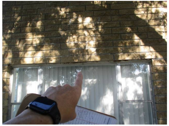
18 Right Side 1st Floor Lintel Severe Corrosion w/ Sag
