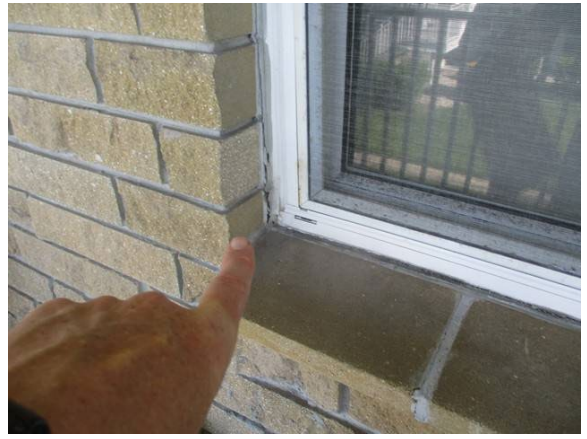
10 Caulking Deteriorated/Missing Windows Throughout
