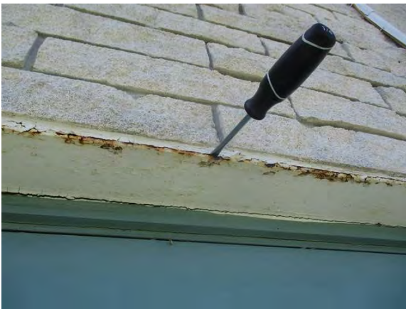
29 Rear of Building Lintel Sag w/ Severe Corrosion
