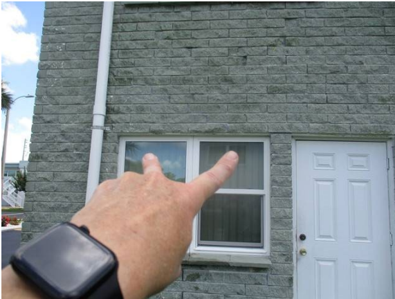
19 Rear of Building Lintel Sag w/ Severe Corrosion
