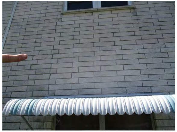
42 Rear of Building Fluted Block Cracked Between 1st & 2nd Floor
