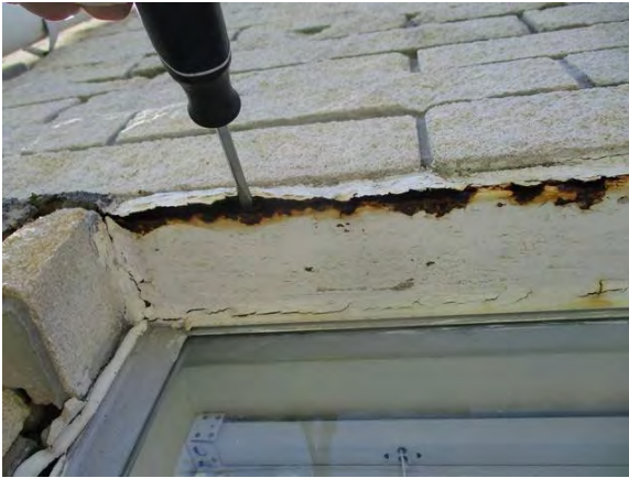
27 Rear of Building Lintel Sag w/ Severe Corrosion
