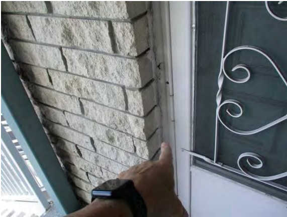
11 Door Caulking Deteriorated/Missing Throughout
