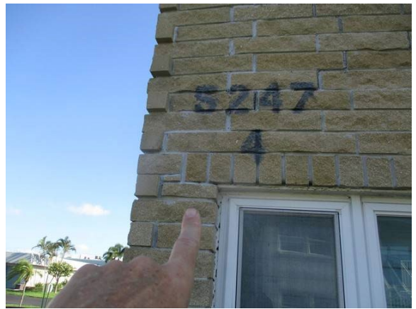
14 Front Left Lintel Sag w/ Excessive Corrosion Fluted Block Cracking
