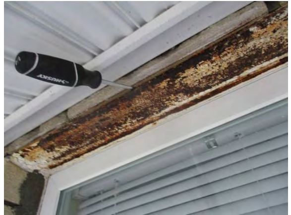
6 Front Left Lintel Sag w/ Severe Corrosion
