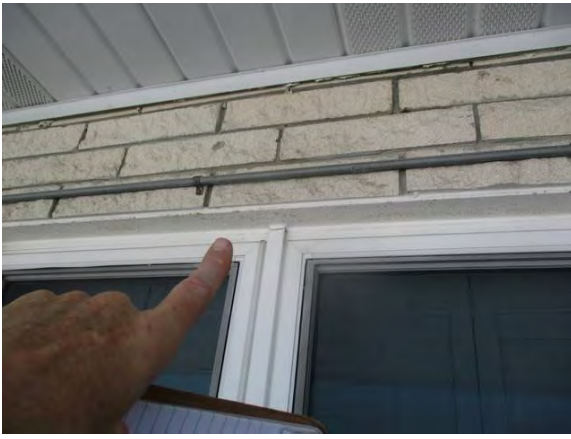
9 2nd Floor Walkway Lintels Minor Corrosion
