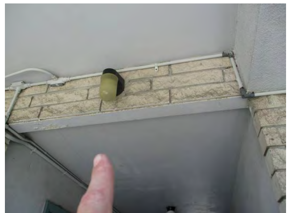
16 Hallway Lintel Minor Corrosion/Peeling Paint
