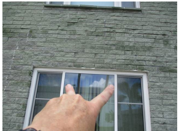
16 Right Side of Building Lintel Sag
