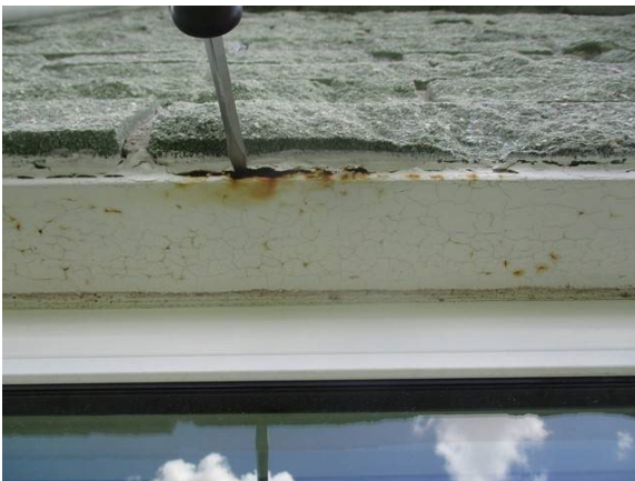
21 Rear of Building Lintel Sag w/ Severe Corrosion
