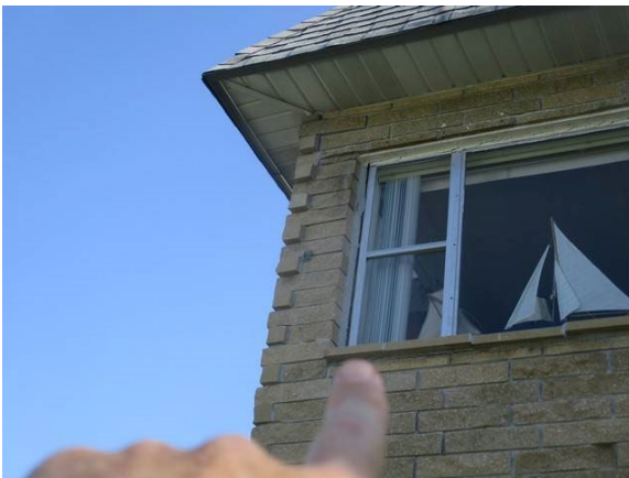
15 Front Left 2nd Floor Window Separation
