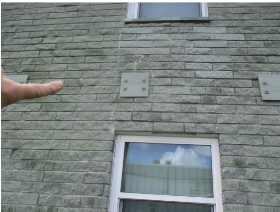
15 Right Side of Building Fluted Block Cracked Between 1st & 2nd Floors
