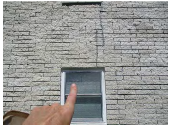
18 Right Side of Building Lintel Sag w/ Severe Corrosion
