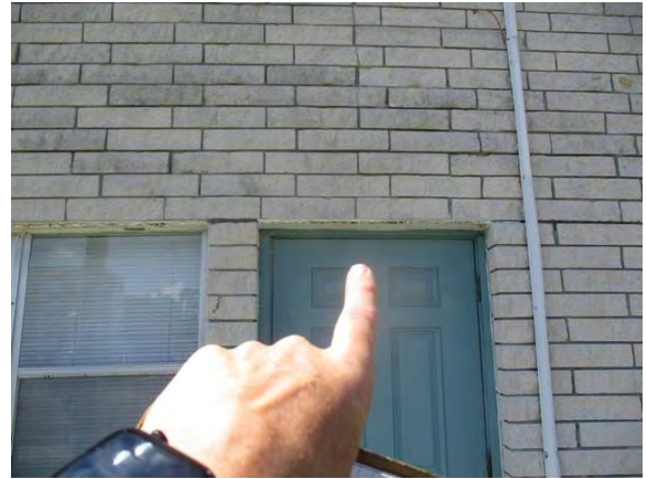
28 Rear of Building Lintel Sag w/ Severe Corrosion
