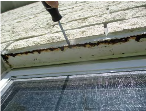
21 Right Side of Building Lintel Sag w/ Severe Corrosion
