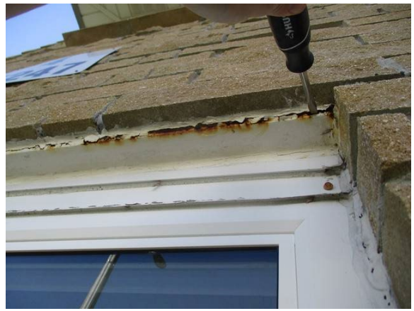
50 Left Side of Building Lintel Sag w/ Severe Corrosion
