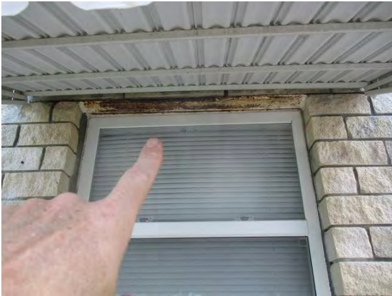
5 Front Left Lintel Sag w/ Severe Corrosion
