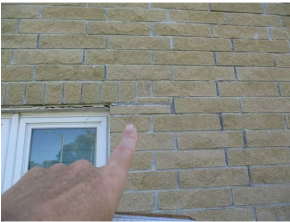
13 Front Left Lintel Sag w/ Excessive Corrosion Fluted Block Cracking
