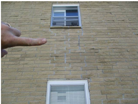
53 Left Side of Building Fluted Block Cracking Between 1st & 2nd Floor
