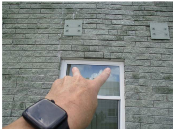
14 Right Side of Building Lintel Sag w/ Severe Corrosion
