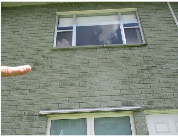
25 Rear of Building Fluted Block Cracked Between 1st & 2nd Floors
