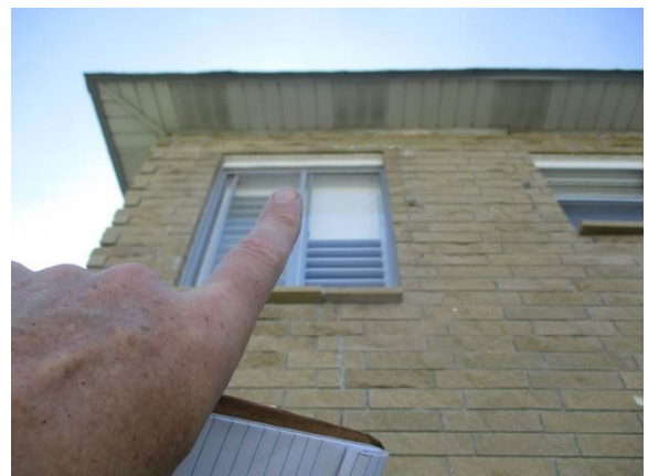
48 Left Side of Building 2nd Floor Lintels Minor Corrosion
