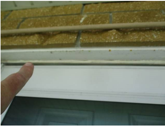
9 Lintels 2nd Floor Walkway Minor Corrosion
