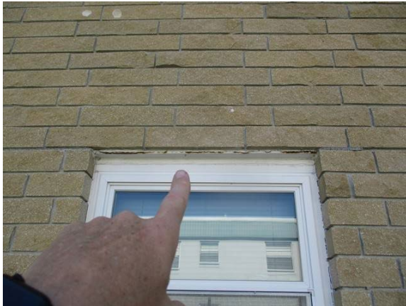
51 Left Side of Building Lintel Sag w/ Severe Corrosion
