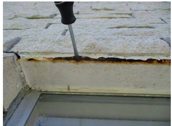
32 Rear of Building Lintel Sag w/ Severe Corrosion
