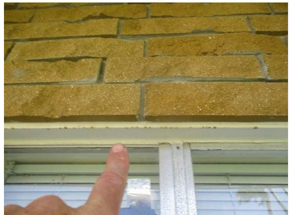
16 Lintels 1st Floor Walkway Minor Corrosion
