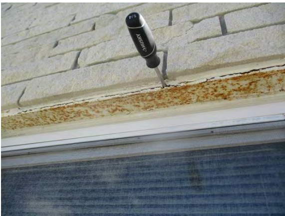
13 Front Right Lintel Sag w/ Severe Corrosion
