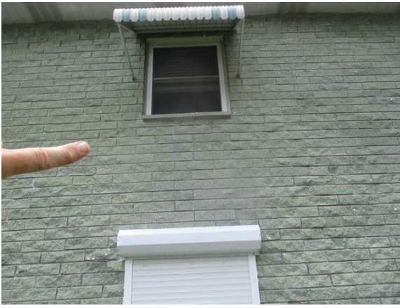
49 Left Side of Building Fluted Block Cracked Between 1st & 2nd Floors
