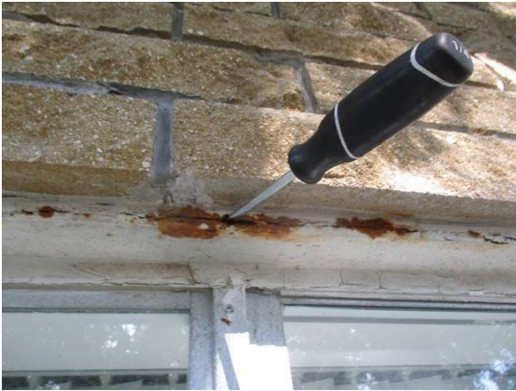
19 Right Side 1st Floor Lintel Severe Corrosion
