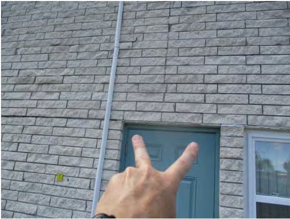
35 Rear of Building Lintel Sag w/ Severe Corrosion
