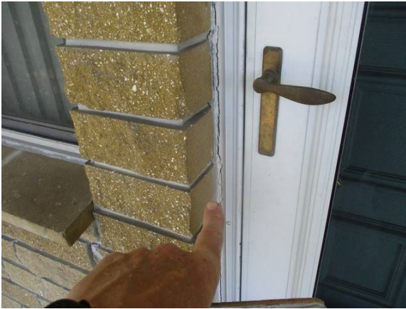
11 Caulking Deteriorated/Missing Doors Throughout
