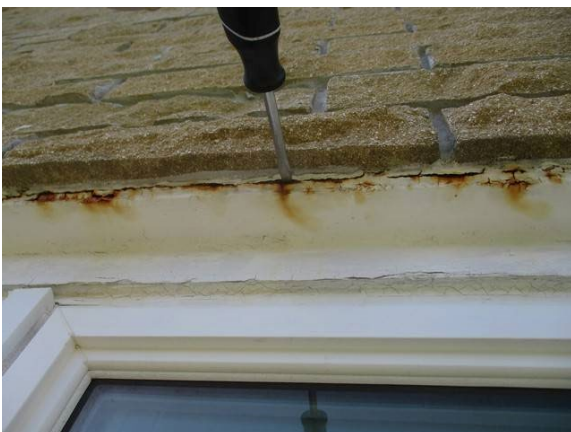
47 Rear of Building Lintel Sag w/ Severe Corrosion
