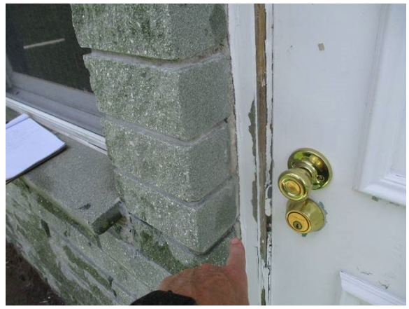
34 Door Caulking Deteriorated/Missing Throughout
