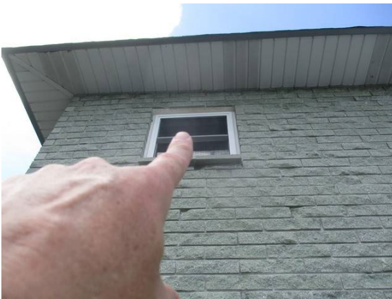
5 2nd Floor Lintels Minor Corrosion
