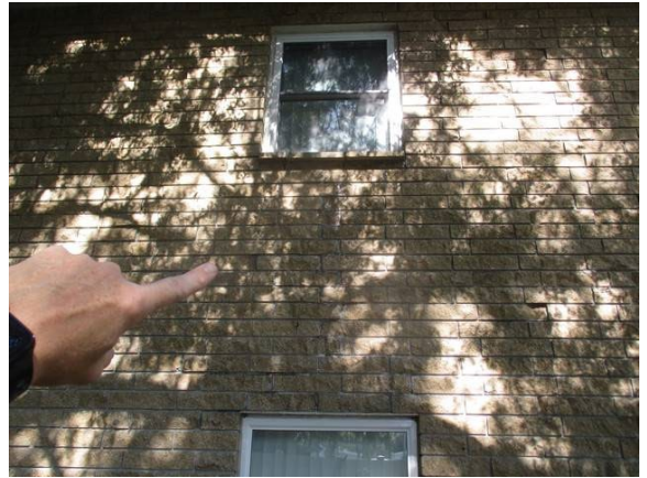
20 Right Side 1st Floor Lintel Severe Corrosion w/ Sag & Fluted Block Cracks
