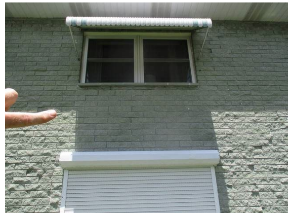
48 Left Side of Building Fluted Block Cracked Between 1st & 2nd Floors
