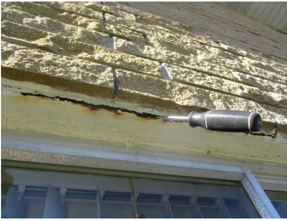
25 Rear of Building Lintel Severe Corrosion w/ Sag
