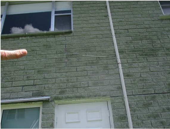
27 Rear of Building Fluted Block Cracked Between 1st & 2nd Floors
