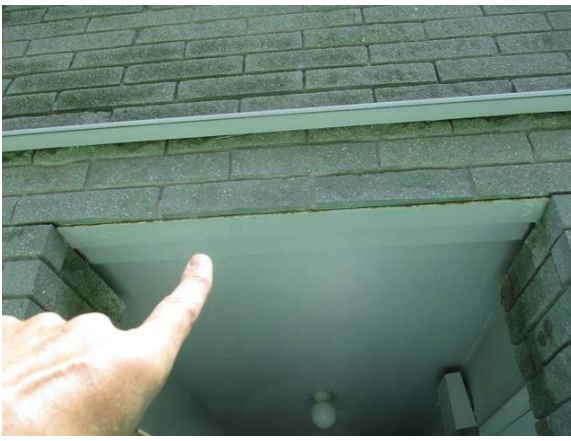
41 Hallway Lintel Minor Corrosion
