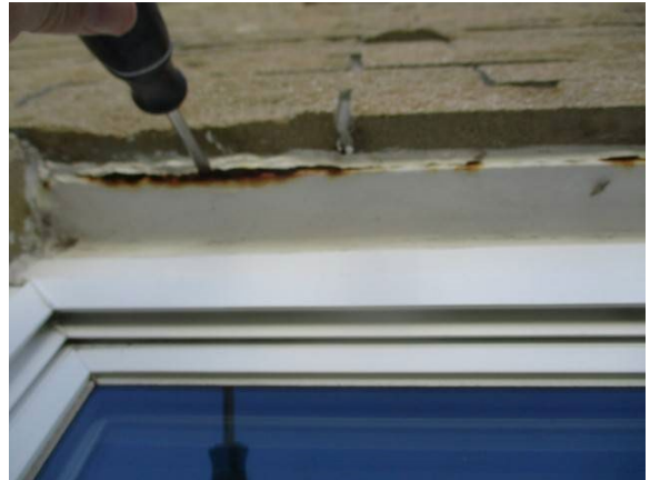
52 Left Side of Building Lintel Sag w/ Severe Corrosion
