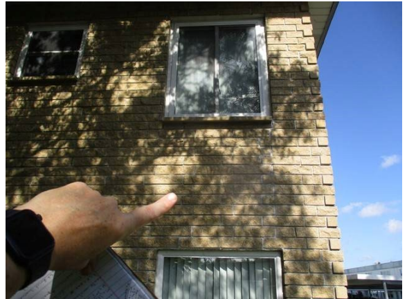
22 Right Side 1st Floor Lintel Severe Corrosion w/ Sag & Fluted Block Cracks
