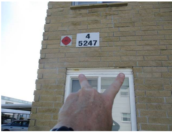
49 Left Side of Building Lintel Sag w/ Severe Corrosion
