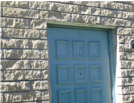
29 Rear of Building Lintel Severe Corrosion w/ Sag
