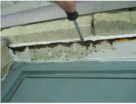
41 Rear of Building Lintel Sag w/ Severe Corrosion
