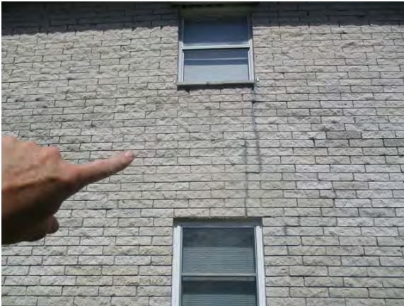
19 Right Side of Building Fluted Block Cracked Between 1st & 2nd Floors
