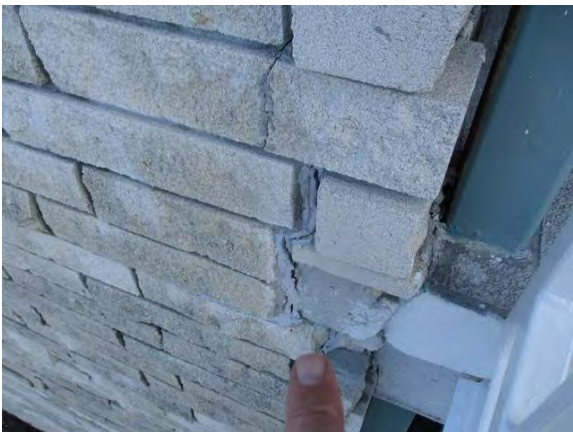
7 Front Left Fluted Block Cracking Between 1st & 2nd Floors
