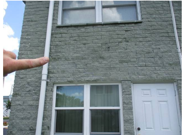
20 Rear of Building Fluted Block Cracked Between 1st & 2nd Floors
