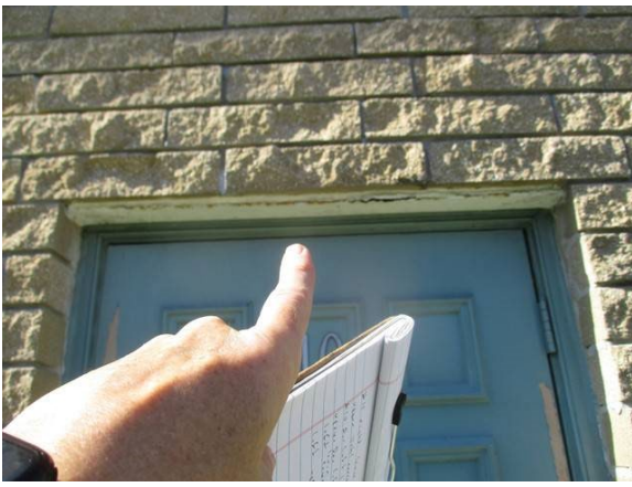
33 Rear of Building Lintel Severe Corrosion w/ Sag
