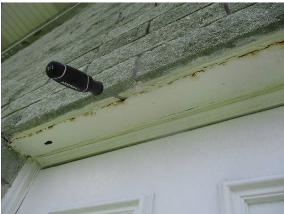
37 Rear of Building Lintel Sag w/ Severe Corrosion
