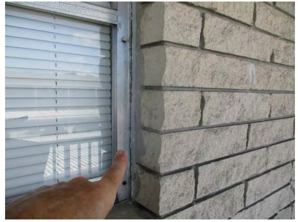
10 Window Caulking Deteriorated/Missing Throughout
