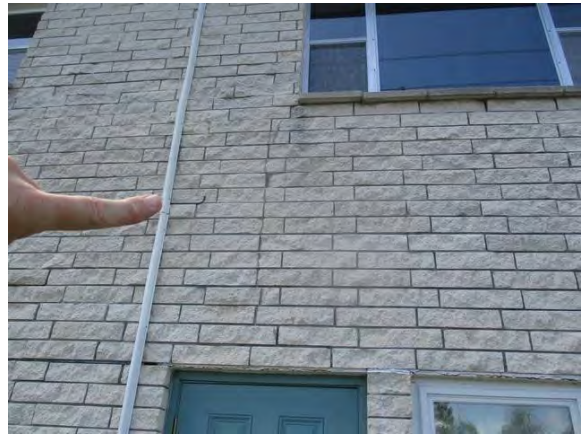
34 Rear of Building Fluted Block Cracked Between 1st & 2nd Floor
