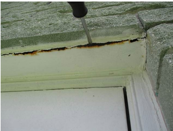
31 Rear of Building Lintel Sag w/ Severe Corrosion
