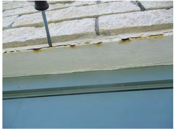
36 Rear of Building Lintel Sag w/ Severe Corrosion
