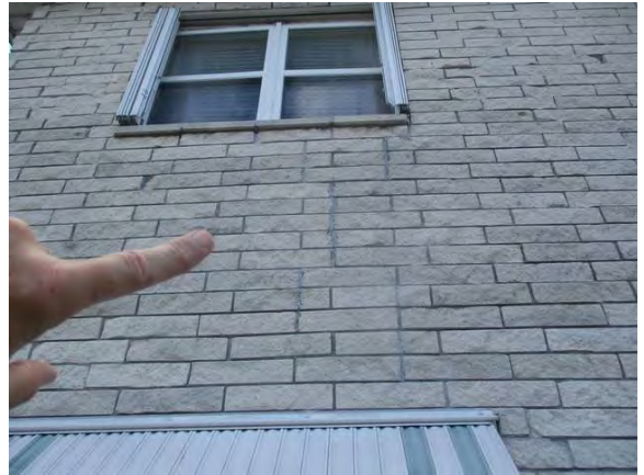
52 Left Side of Building Fluted Block Cracked Between 1st & 2nd Floor
