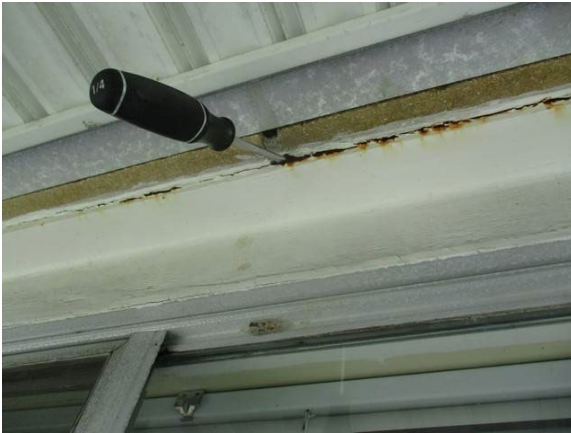
43 Rear of Building Lintel Sag w/ Severe Corrosion
