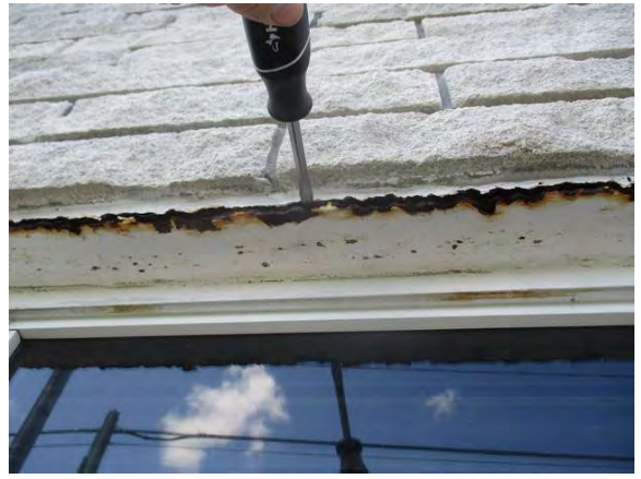
50 Rear of Building Lintel Sag w/ Severe Corrosion
