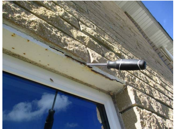
28 Rear of Building Lintel Severe Corrosion w/ Sag
