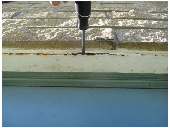
34 Rear of Building Lintel Severe Corrosion w/ Sag
