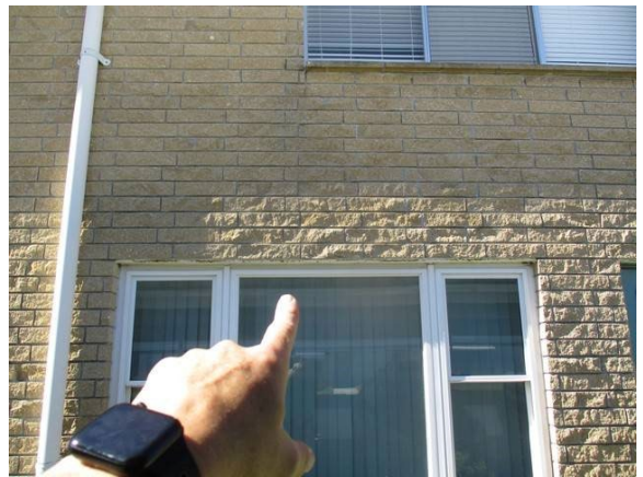
30 Rear of Building Lintel Severe Corrosion w/ Sag
