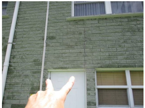
30 Rear of Building Lintel Sag w/ Severe Corrosion
