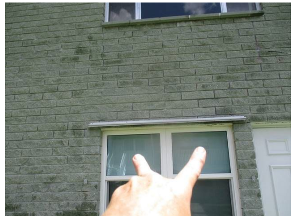
24 Rear of Building Lintel Sag w/ Severe Corrosion
